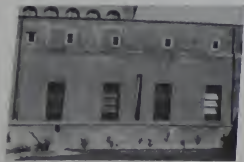
FIG. 77. B. Stubbins. Facade of narthex.
